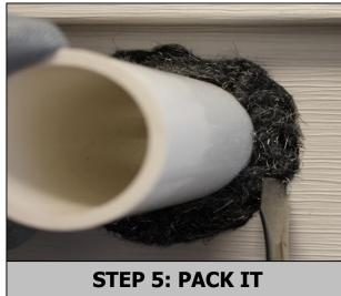
Using the blunt side of a screwdriver, push the material into the opening so that it is flush to, or slightly below the surface of the opening. Properly installed, *Xcluder* will expand to form a better seal shortly after installation.
